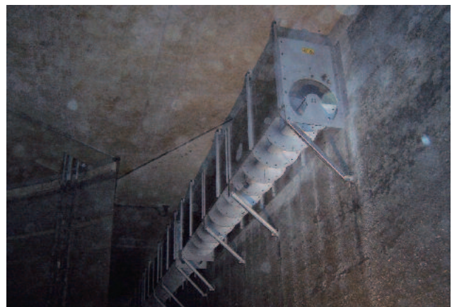
View of the upstream side and lateral screenings discharge opening
